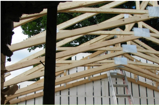
View of scissor trusses used in rear addition
