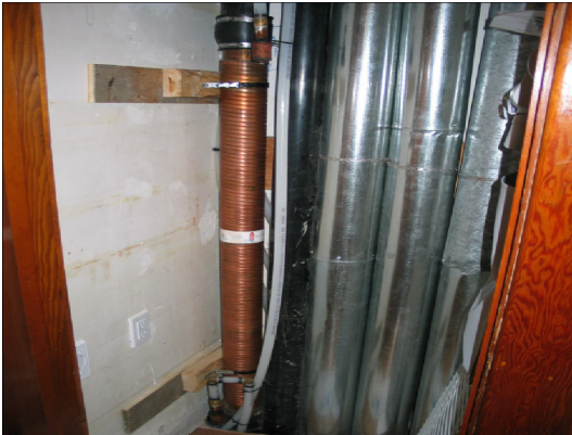
The waste water copper heat exchanger (shown left of ductwork) is contained in a closet on the main floor. The bathrooms are upstairs and connected to the grey water system in the basement.
