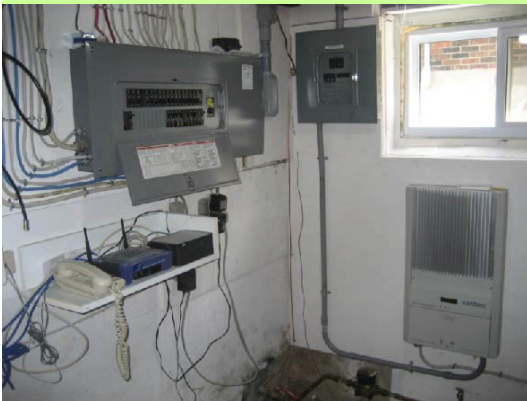
Layout of electrical equipment, showing the grid tied inverter which supplies electricity to the meter located just outside the window.
