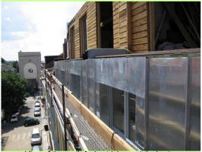
View of the north-facing triplex and duplex terraces. Part of the wall already has a zinc finishing.
