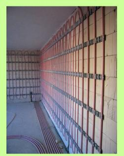
Silicate block wall and surface heating tubing.
