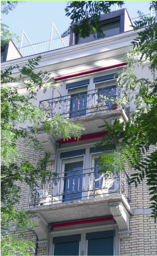
The street façade could not be changed
