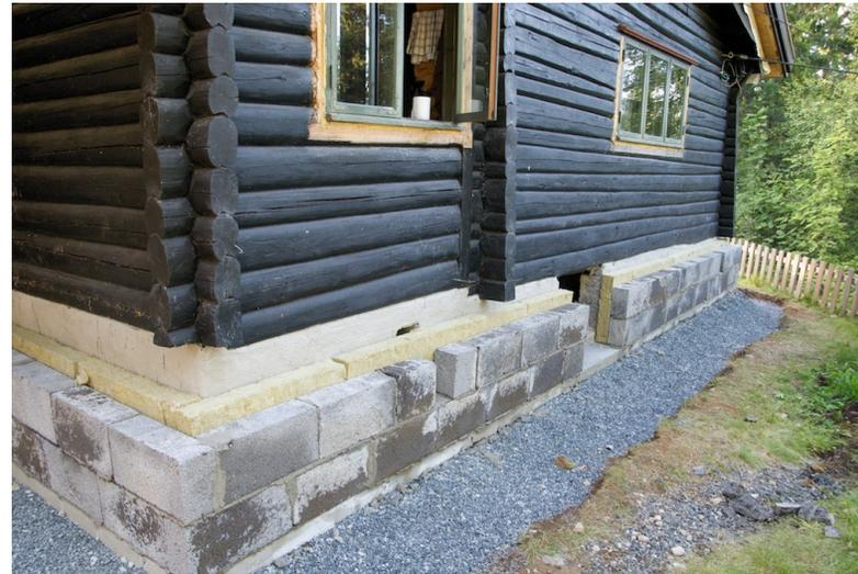
The floor of the crawl space is covered with a 0.2 mm moisture barrier, then 150 mm insulation. Foundation walls are insulated with 100 mm mineral wool and 70 mm edge insulation. The crawl space is sealed to keep the temperature above the condensation point (temperature and humidity will be monitored).
