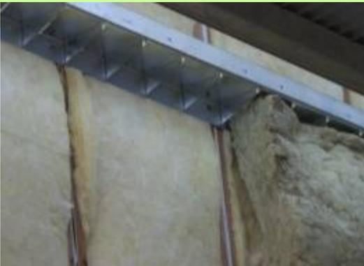
After removing the panels and old insulation of the gable walls, 2 layers of insulation were added.
