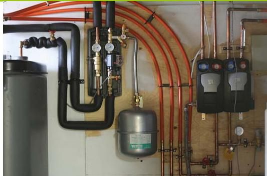
Regular natural gas domestic hot water tanks (DHW) have an efficiency range of 55-60%. The Now House employs a compact wall-hung high efficiency boiler which improves efficiency to above 90%. This gas boiler provides heat only when necessary (to the solar storage tank) as a back up to the solar thermal system.
